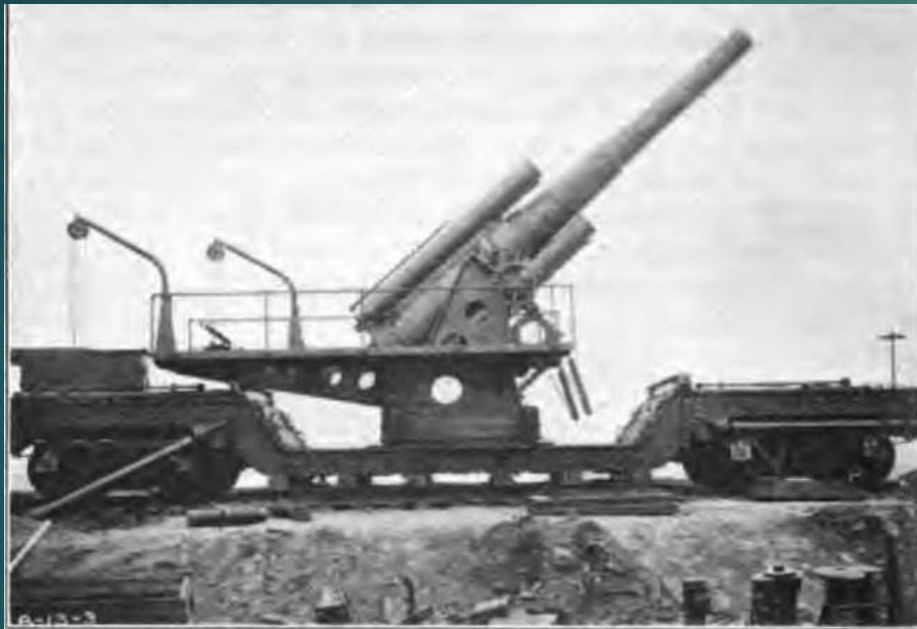
FIG. 31.—8-inch railway mount, model of 1918, showing firing platform formed by crossties laid on H-beams.
